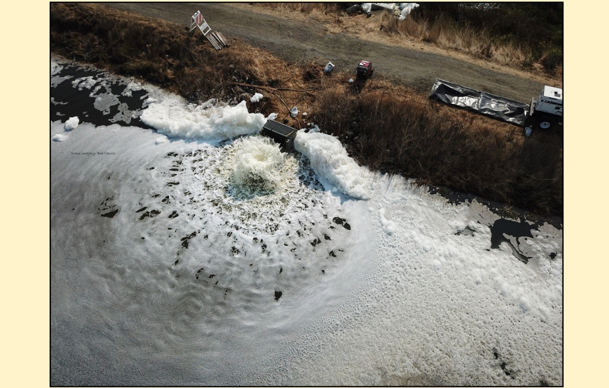
Fig.: After sediment settles, water is aerated before being released back to the river to meet water regulations.
